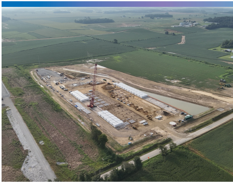
BESS yard and substation: Battery units are onsite and ready for installation, and substation foundation has been completed ahead of transformer delivery.
