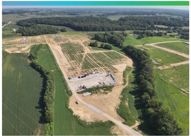
Laydown number 1: Piles are installed and tracker layout just starting.
