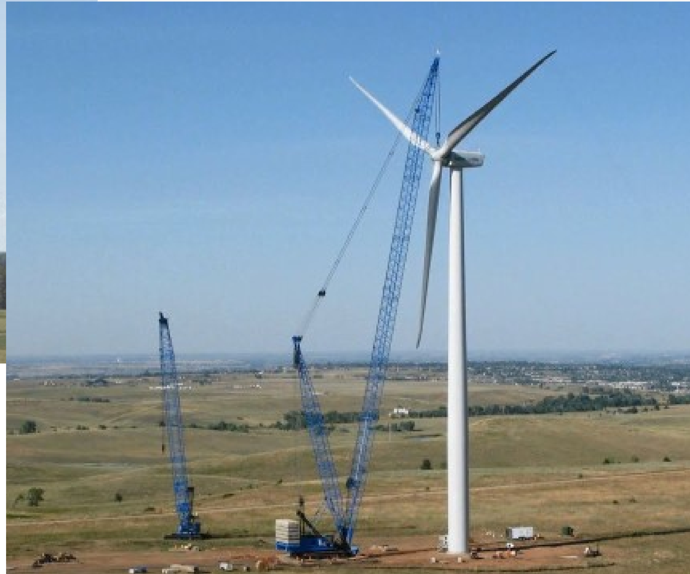
New Rotor Installation
