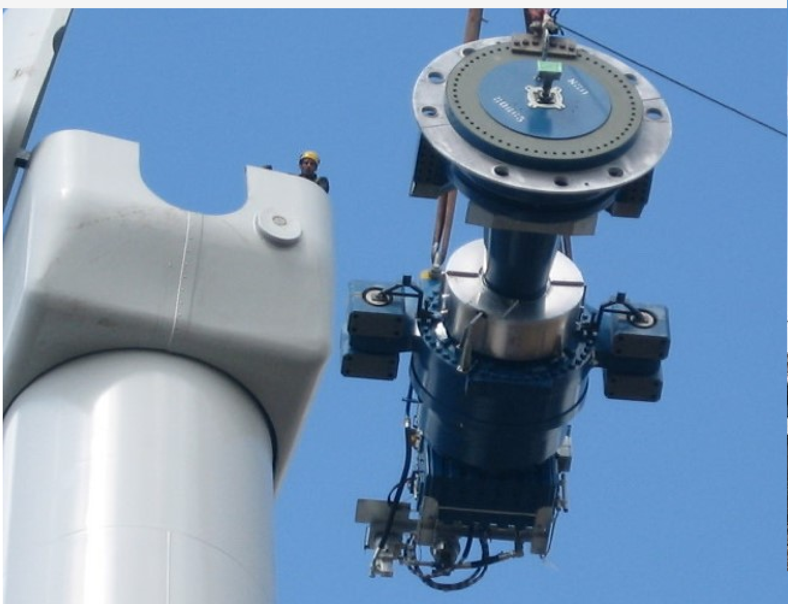
New Drivetrain Installation
