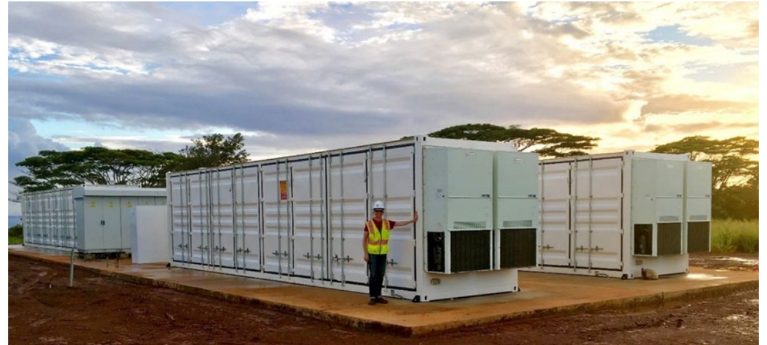
Containerized Lithium-Ion Batteries
