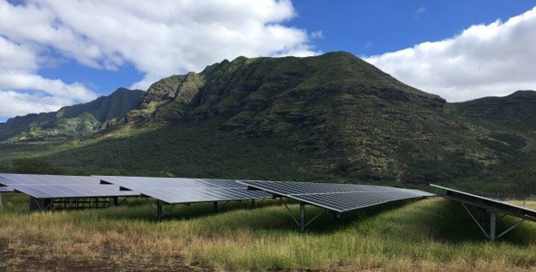
Photovoltaic Panels and Racking System
