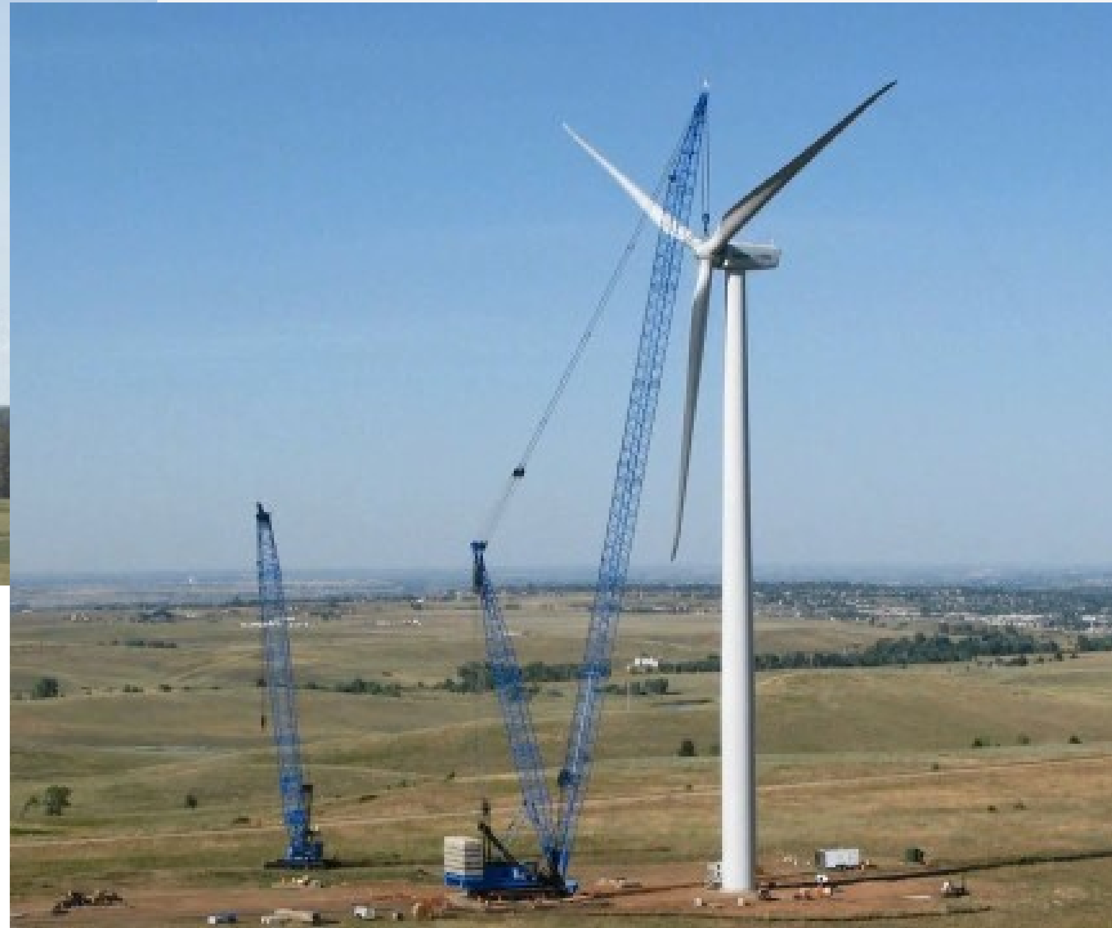
New Rotor Installation
