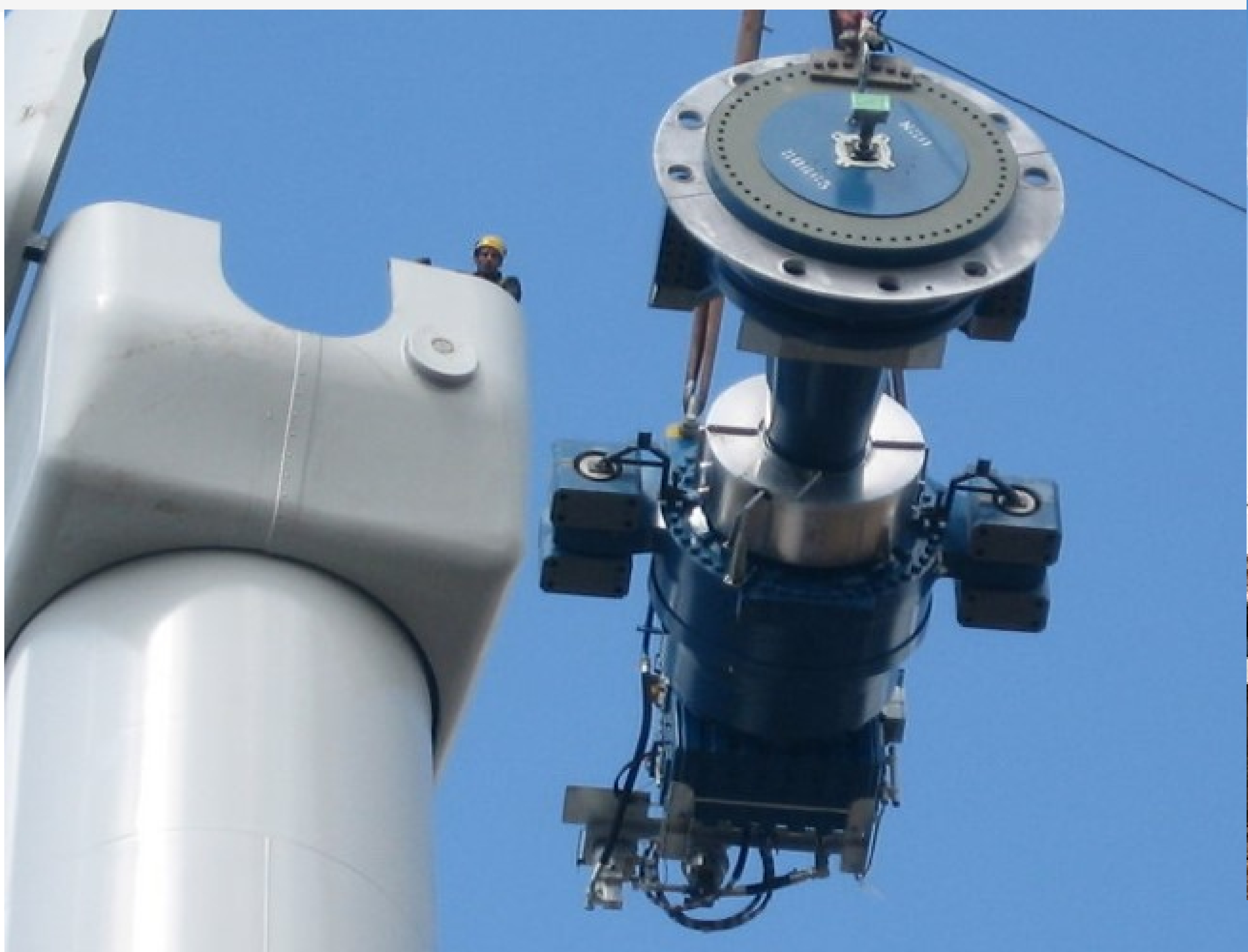
New Drivetrain Installation
