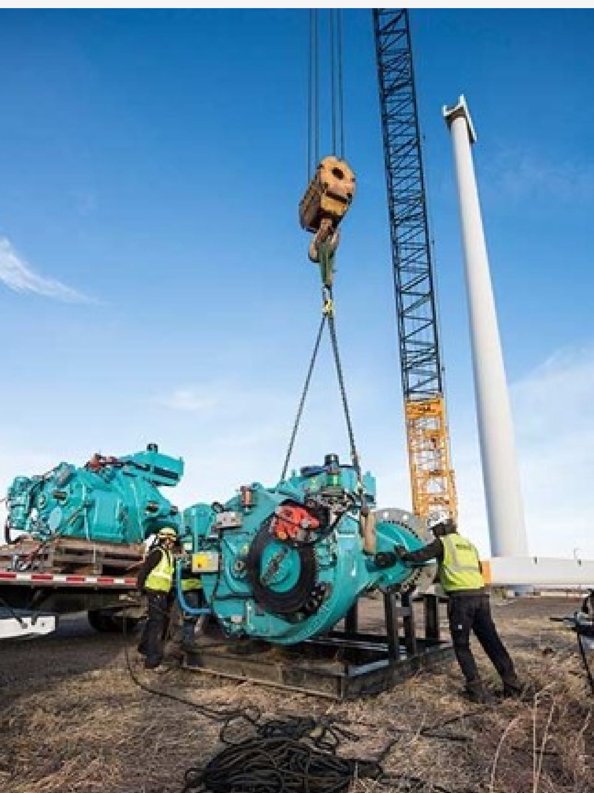
New Drivetrain Installation
