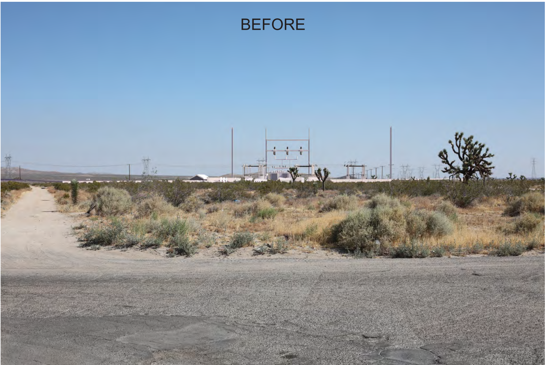
a) View to the north from Muskrat Avenue at El Mirage Road. Substation and BESS Yard Location Alternative A, which was approved as part of the Baldy Mesa Solar Project, is visible to the north.
