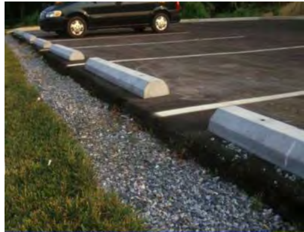
Fig 2.2c. Gravel Diaphragm
