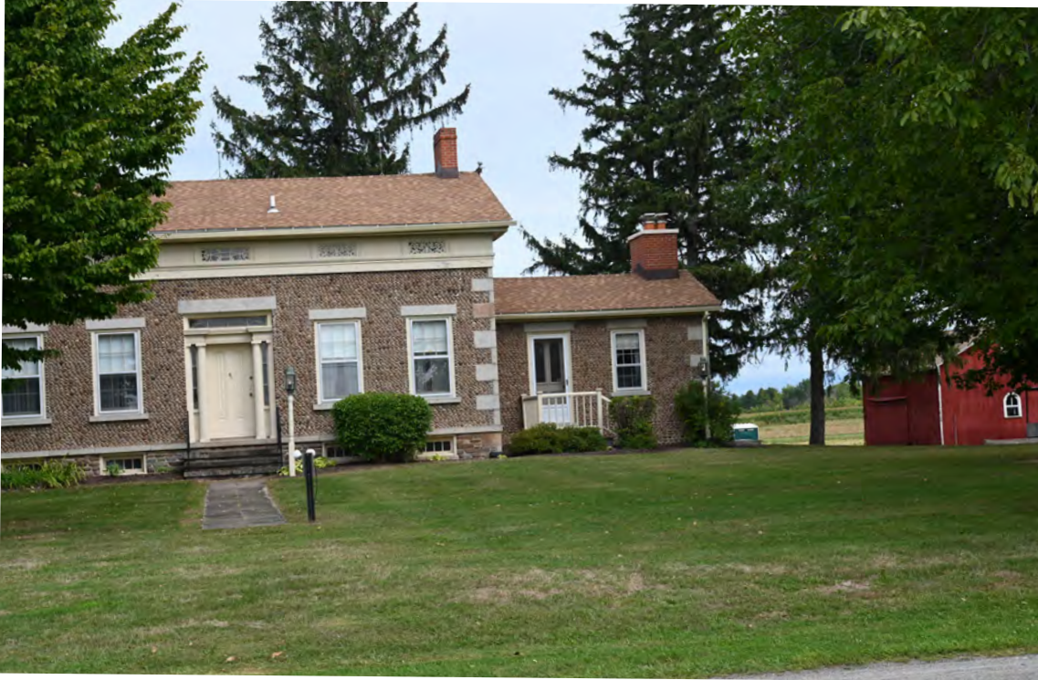
Looking north from NY-18/Lake Rd. toward front of Babcock House
