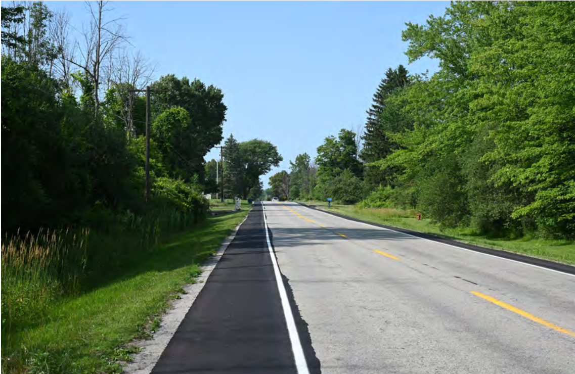
Looking North from Hartland Rd at entry of Niagara Hartland RV resort. Leaf on season viewing condition.
