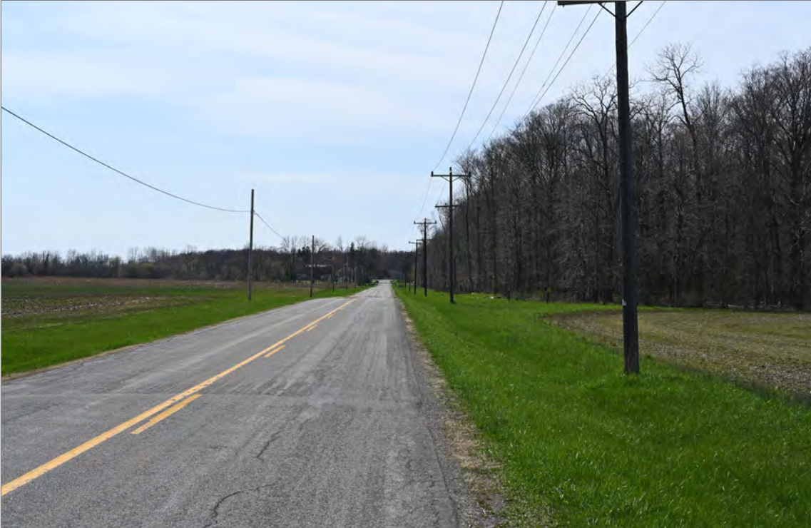
Looking west along Haight Road.
