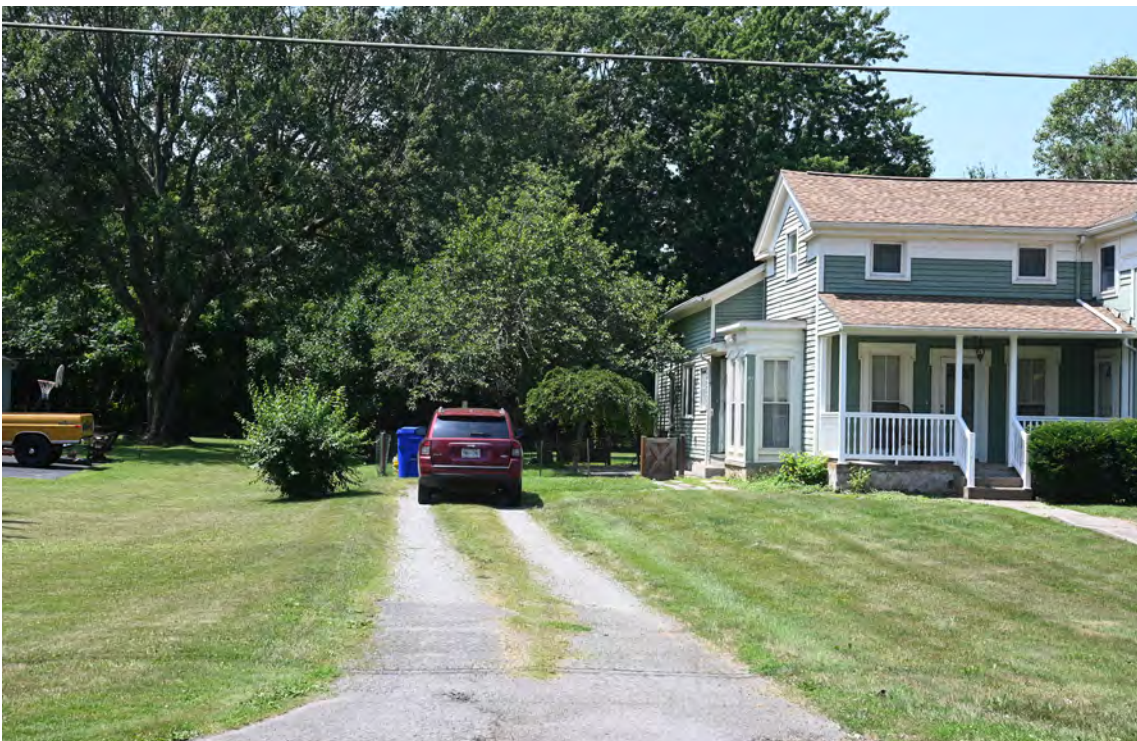
Looking West toward project area from Quake Rd. Leaf on season viewing condition.
