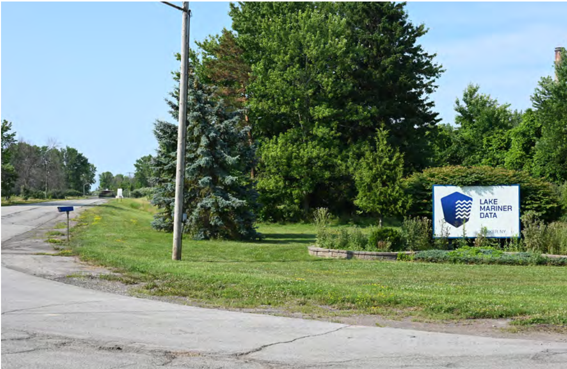
Looking Northeast on Lake Rd toward substation area. Leaf on season viewing condition.
