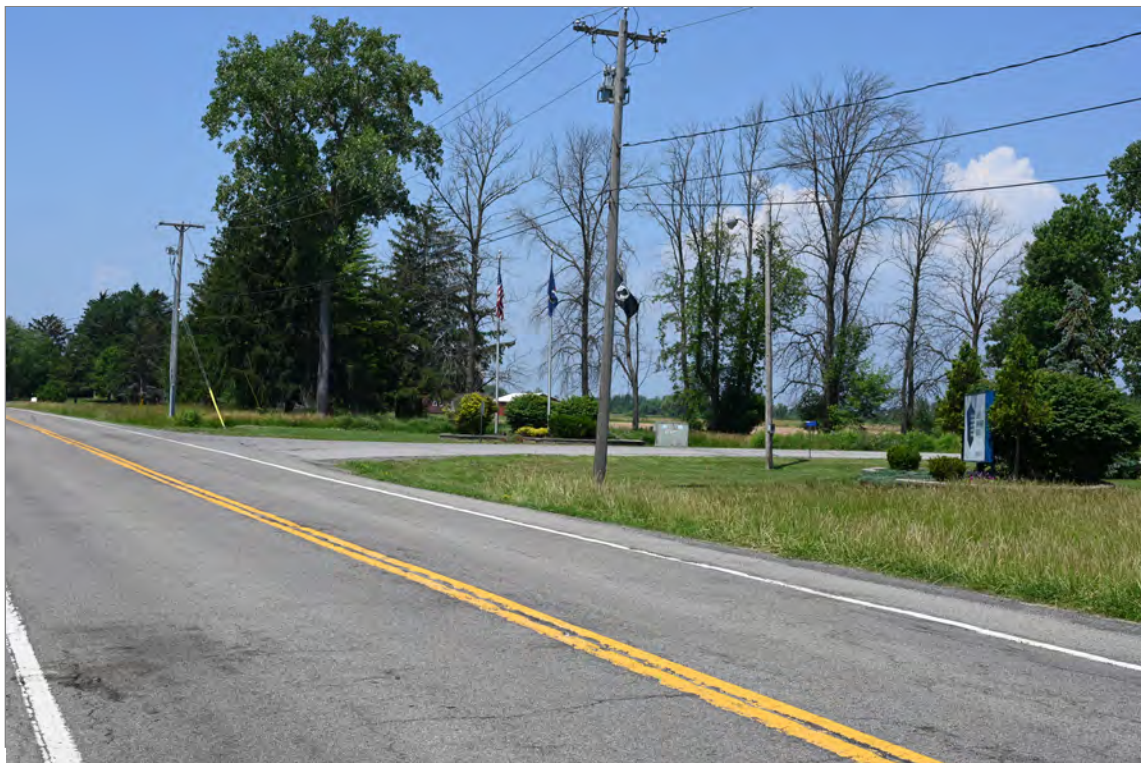
Looking northwest on Lake Road toward entry drive to existing power plant. Leaf off season viewing condition.
