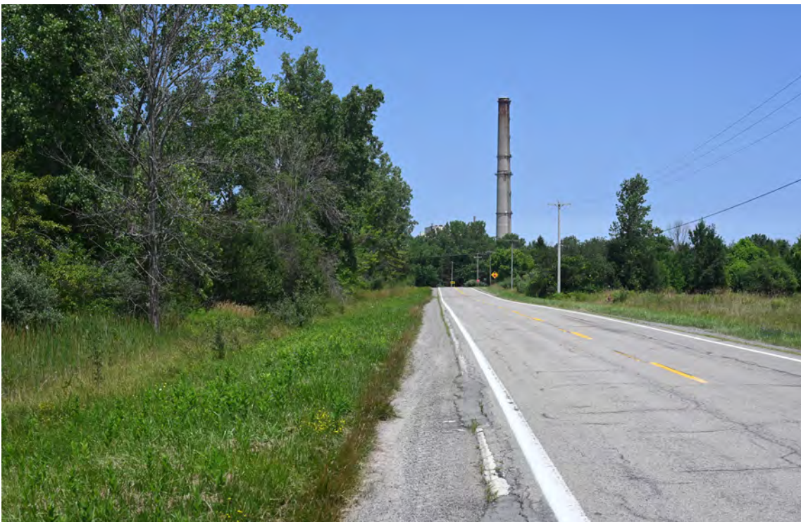
Looking North on Hosmer Rd. Leaf on season viewing condition.
