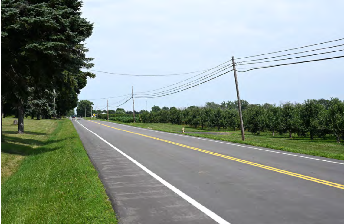
Looking East to project area from North side of Lake Rd. Leaf on season viewing condition.
