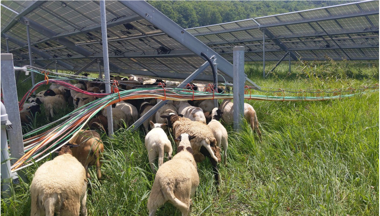
Figure 3. Sheep passing under CAB cabling.
