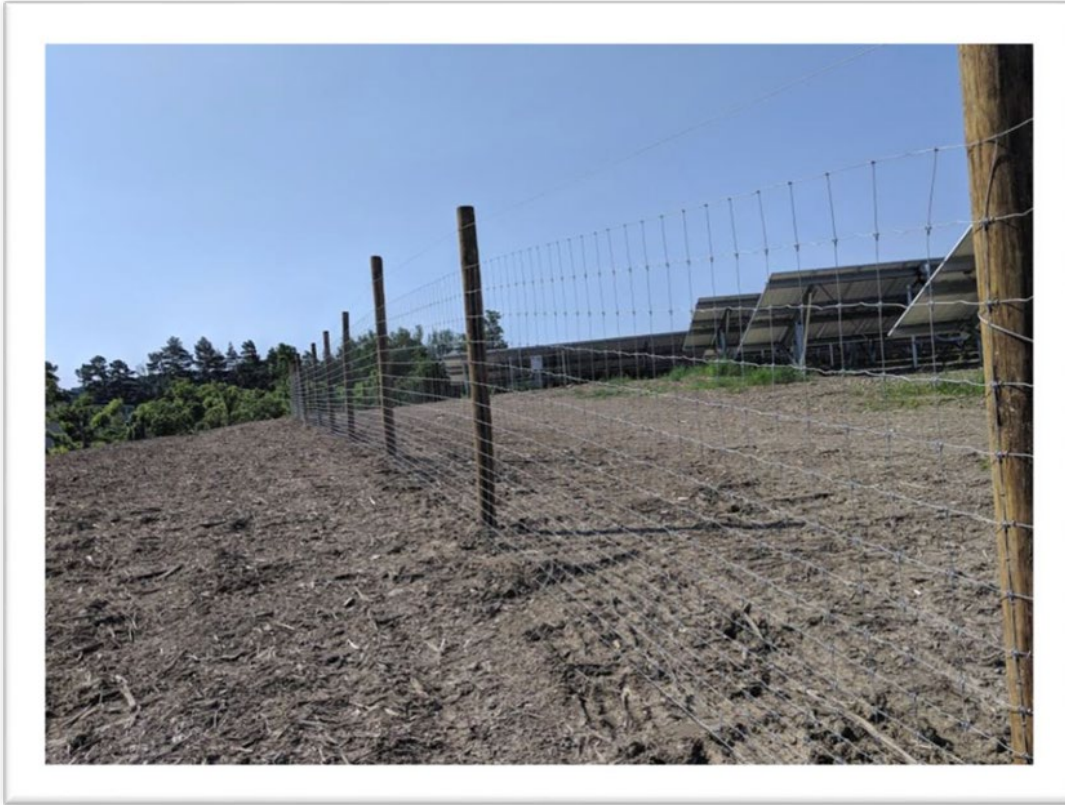
Figure 1. Perimeter fencing that follows grade well.
